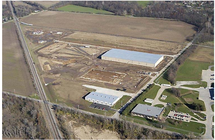
A privately held park, green field sites can be purchased for development for new industrial structures. Rail is located in the FHBP.
