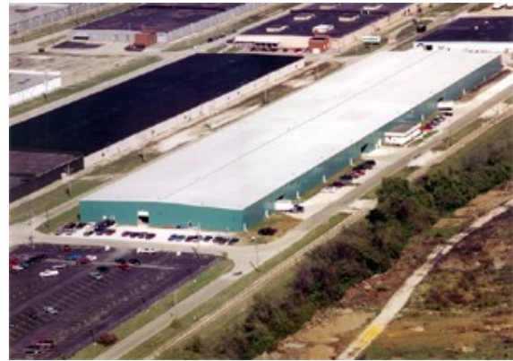
The Everhart Building is adjacent to Fruitridge Avenue with Sony DADC and Bemis as two neighboring industries.
